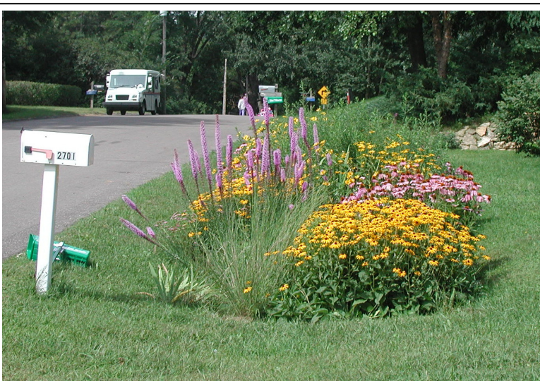
Figure 4.6 Example of a rain garden using native plant species installed in a roadside swale in a residential development. (Source: Minnesota DNR)
