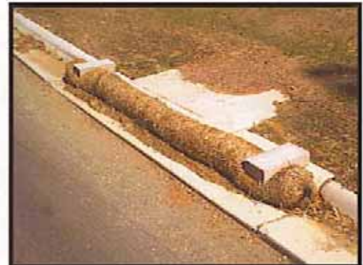
Fig. 14—Storm drain inlet protection
